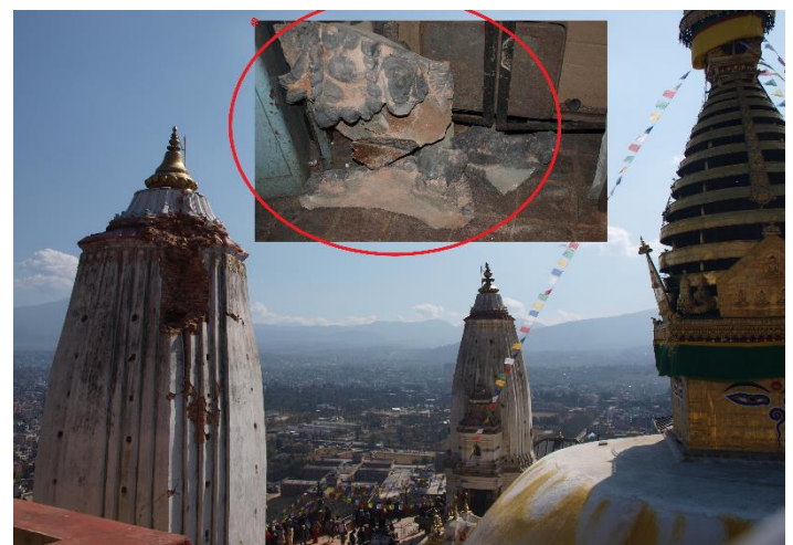
Figure 3: The damaged Pratappur temple at Swyambhunath along with the main stupa and Anantapur temple. Also, shown in the inset is the damaged stone statue that was placed on one side of the main entrance door of the damaged temple.
