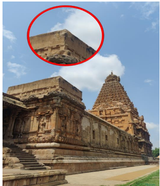
Figure 7: A Photograph of Brihadeeshwara temple located at the bank of the Cauvery river in Tamilnadu India. Shown in the inset is the edge of the temple that was struck by lightning.
