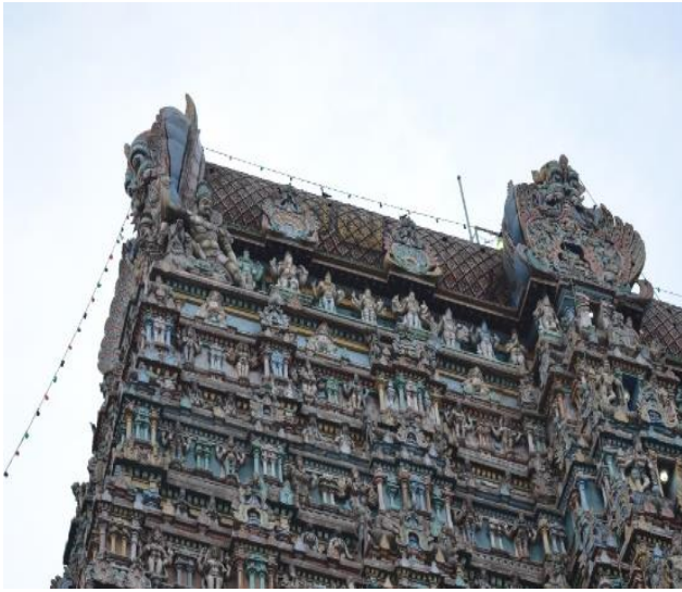
Figure 8: Meenakshi Amman temple located at Madurai Tamilnadu India. An air termination system can be seen on the top of the building.
