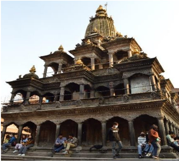
Figure 1: Krishna Mandir (Lord Krishna's temple) built on the premise of Patan Durbar square that has an air termination steeple on the top that is not connected to a down conductor system or an earth termination (to be witnessed).
