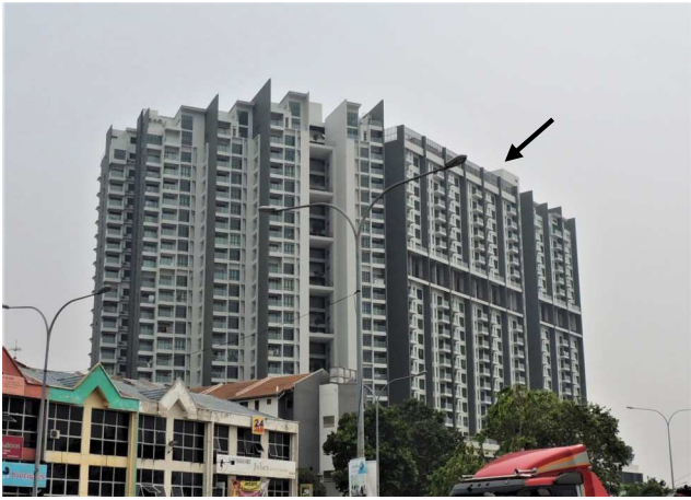
Figure 3 View of UNIV360 Place building from the West showing the location of Bypass #1
