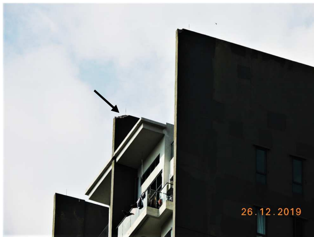
Figure 15 Bypass #9 (Note: Bypass #7 still not repaired)
