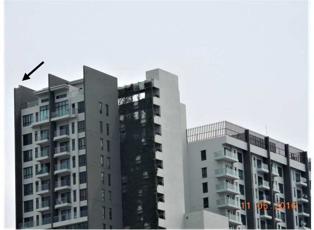
Figure 6 Bypass #3 (Note: Bypass #2 has been repaired)
