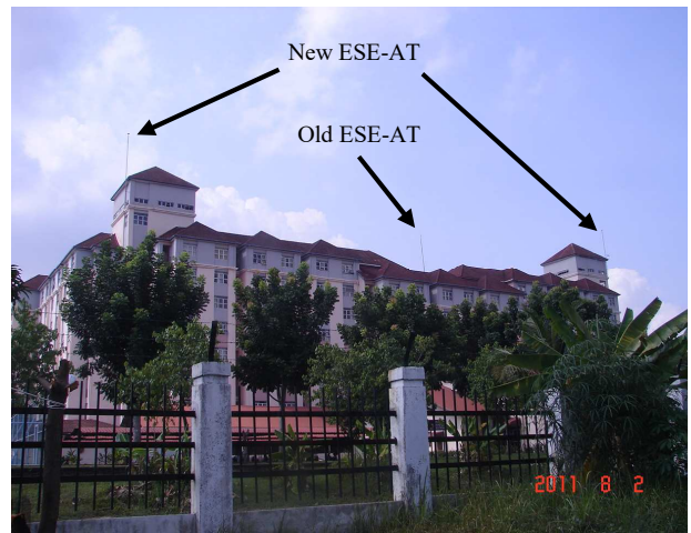
Figure 17 Two new ESE-AT were seen installed at the water tank towers a year later. ( https://goo.gl/maps/kS95jTgfCZs1iLu2A )
