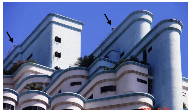
Fig. 4.1. A 100m high apartment building with multi-level roofs installed with two CVM air terminals (arrowed).
