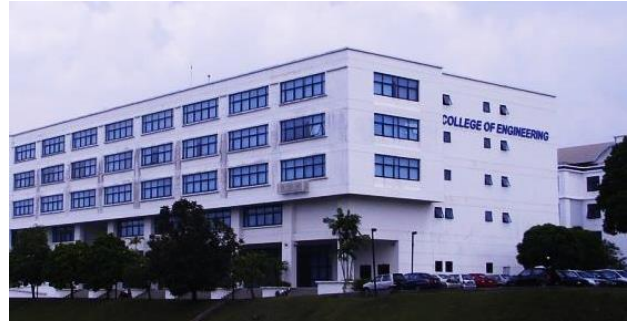
Fig. 4.6. A low-rise college building installed with one ESE and one CVM air terminals.
