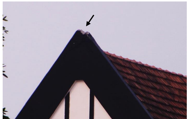
Fig. 2.7. A bypass on top of a pointed facade.
