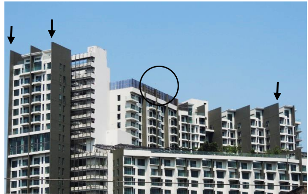
Fig. 3.4. The Univ360 apartment was struck at least six times within a period of two years. The arrows indicate the locations of the major bypasses. See also figs 2.3, 2.4 and 2.5.
