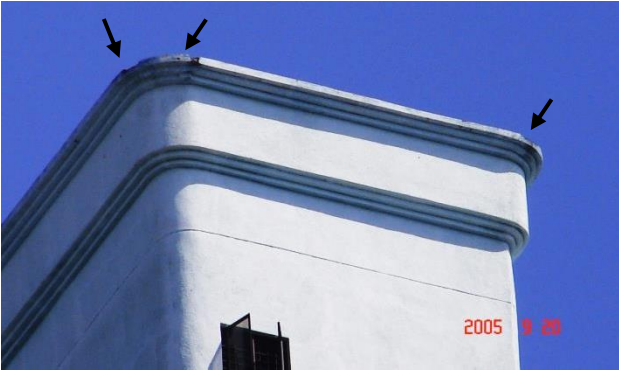
Fig. 4.2. Although located between two CVM air terminals, several bypasses were observed on this section of the upper level roof.
