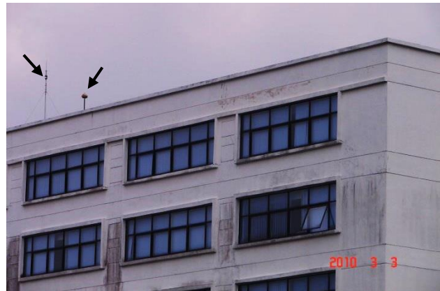
Fig. 4.7. The same building installed with two ESE/CVM air terminals (arrowed) and photographed without a bypass in 2010.
