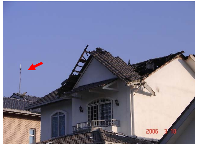
Fig. 2: Close-up view of the ESE air terminal (arrowed) on the adjacent house.
