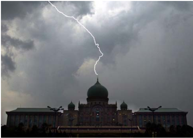
Fig. 8: A photograph of lightning striking the ESE air terminal on the Prime Minister Department building. (Photo credit: The Star Publications plc)
