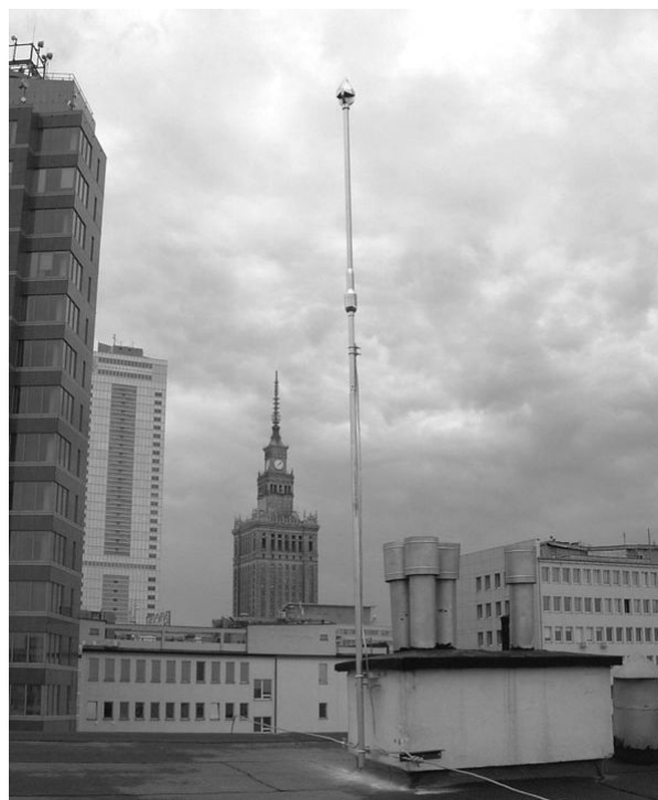
Fig. 3. ESE device in the centre of Warszawa, Poland (photo from the web site of Megatech, one of the ESE sellers)
